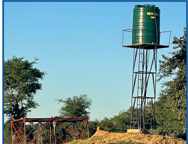
The tank in the background collects water from the solar pump, to be used to irrigate the crops.
